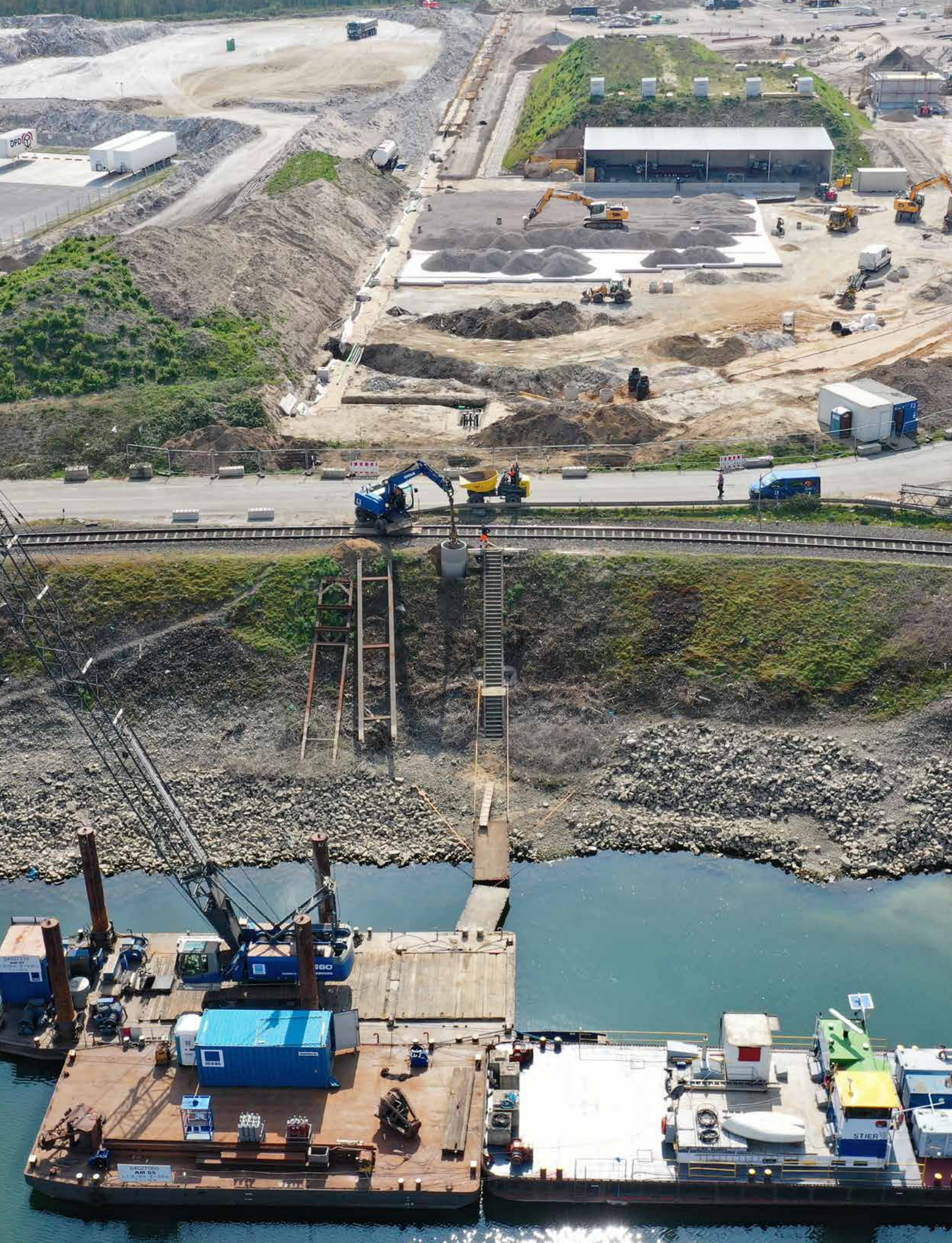
The jetty and rail connection are under development. The site with the already constructed buildings can be seen in the background top right.
